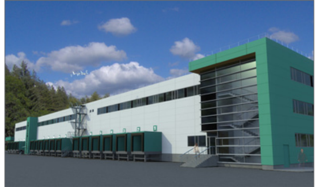
• Transimeksa/Sausupio - new warehousing project on Sausupio Street for particular and market needs.
