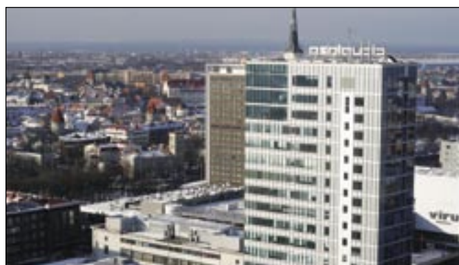
City Plaza, a new 23-storey office building in Central Tallinn.
