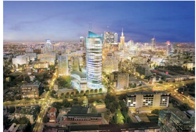
Warsaw Spire, Ghelamco Poland
